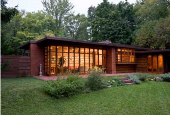
Frank Lloyd Wright Herbert Jacobs House #1 Madison, Wisconsin, 1936–37 Exterior view Photograph by David Heald © The Solomon R. Guggenheim Foundation, New York
